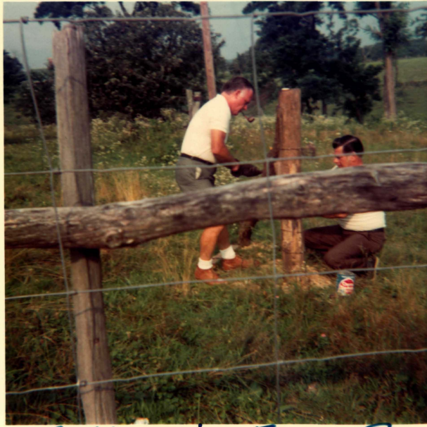
Setting in Fence Posts
